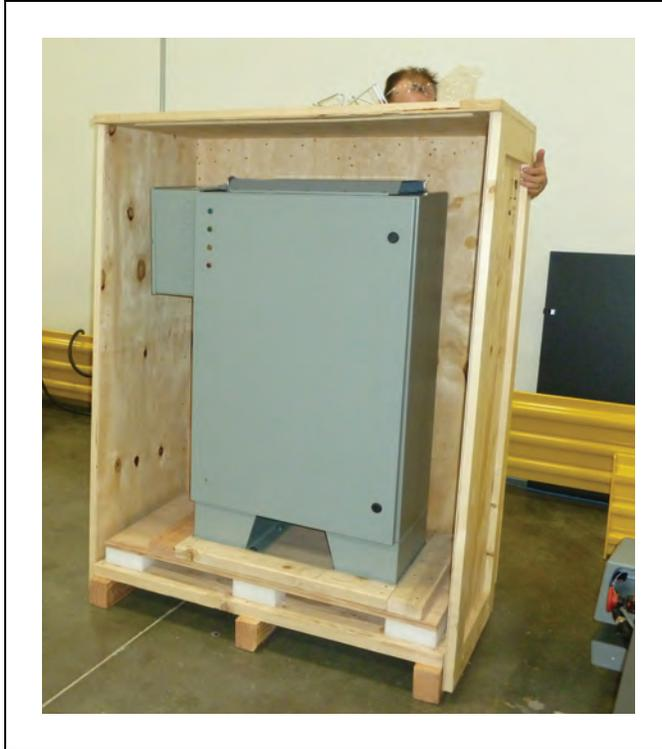
*Figure 3-53. Pulling the Housing Crate Away*
