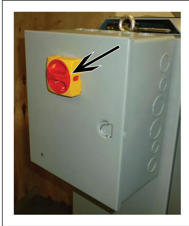
*Figure 8-4. Main Disconnect Switch Placed in OFF Position*
