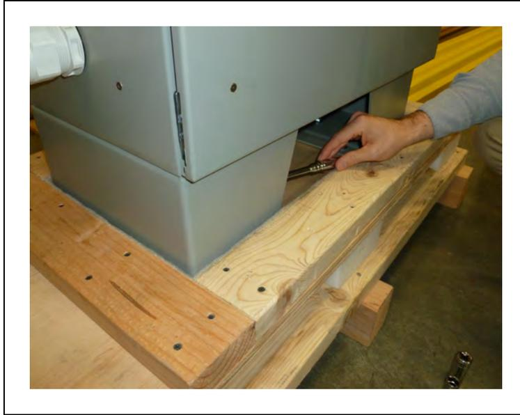
*Figure 3-55. Removing the Bolts Attaching the Power Supply Box to the Base Pallet*
