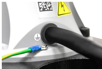
Figure 24: Securing the ground wire with the robot
