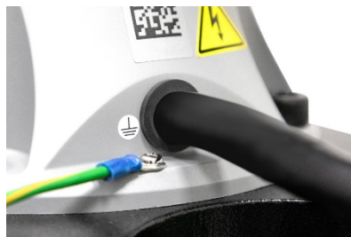
Figure 24: Securing the ground wire with the robot
