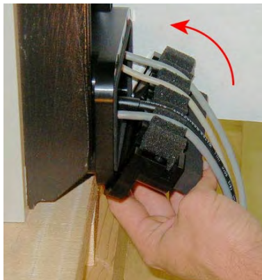
Figure 9-4. Installing Lower Flange
